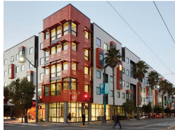
⤴ Nancy and Stephen Grand Family House, San Francisco, USA. 2018. Service d'hébergement. LEED Platinum. @ Leddy Maytum Stacy Architects
