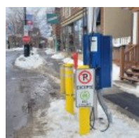
Addition of 4 new electrical
